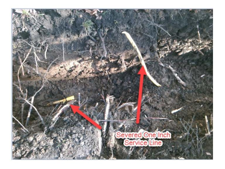
The picture below details the temporarily repaired service line at 729 W Elm Street on 1/6/2020
