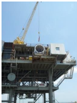
Figure 3. Lifting RTP Spool onto Platform
