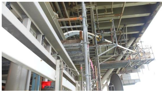
Figure 4. RTP Being Pulled from Platform
