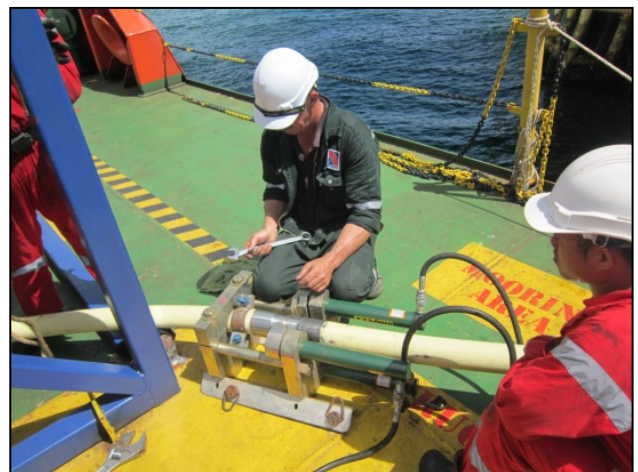
Figure 12: Splicing Lead End on Coupling
