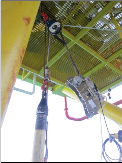
Figure 13: Final Pull Out of the Existing Pipeline
