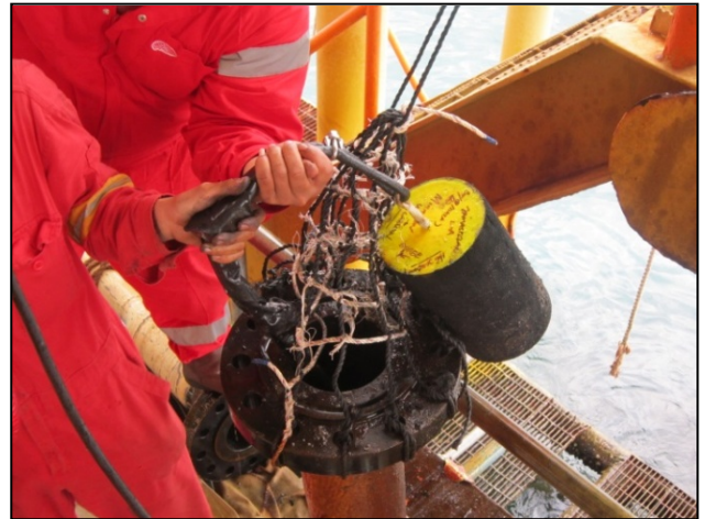
Figure 7: Retrieval of Foam Pig Attached with Pulling Rope
