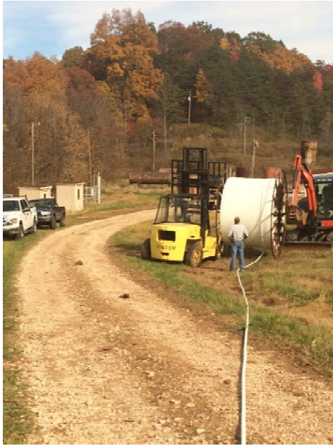
No Special Equipment for Unspooling
