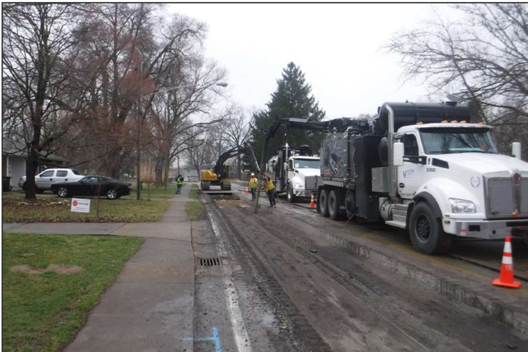
Photograph 4.2. Centerline trench, asphalt removal, West Street, facing south.
