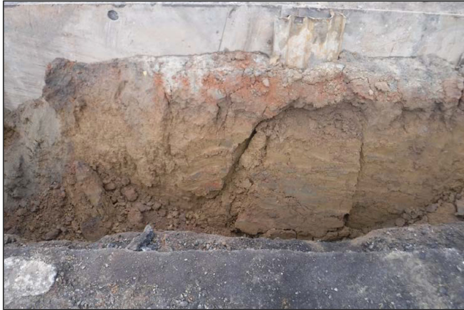
Photograph 4.7. Centerline trench, brick layer and small brick fragments, intersection of West Street and West Pleasant Street.
