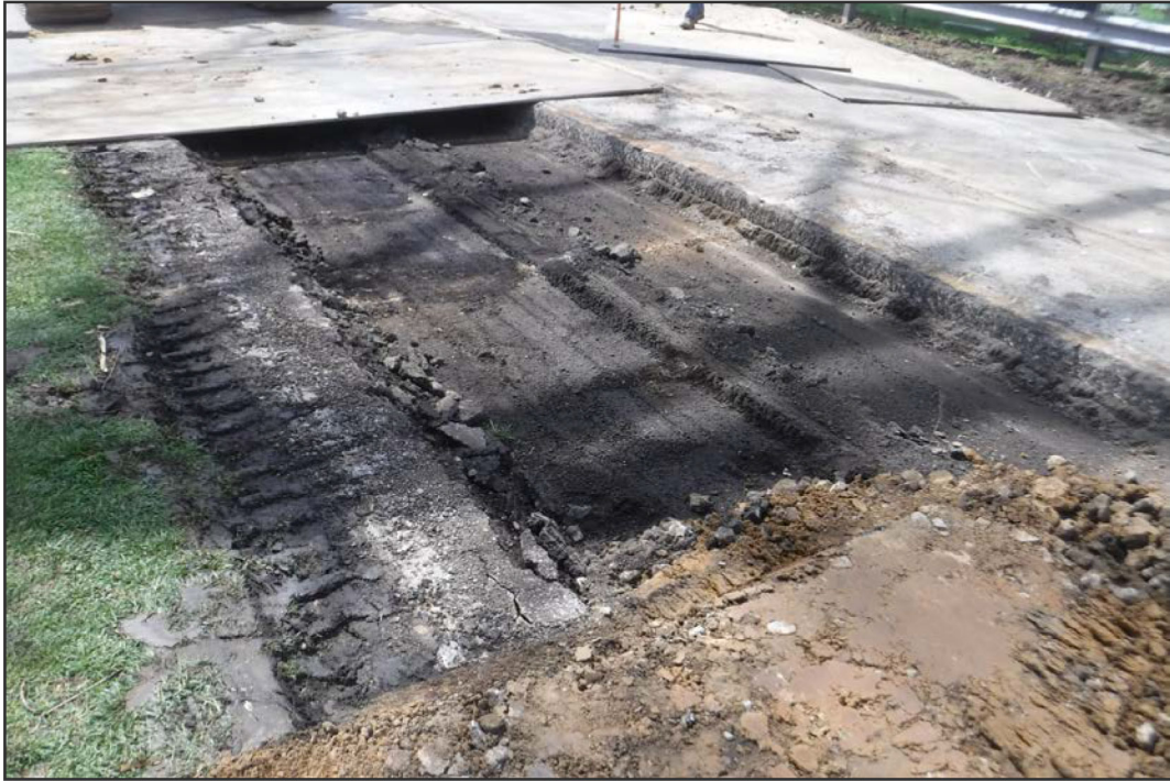
Photograph 4.9. Overview, centerline trench, asphalt removal along Pleasant Street, facing west.
