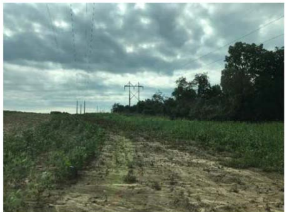
Photograph 4. STR WRO-9615 (3-pole), in distance of ROW. Looking Southeast. (August 8, 2020)
