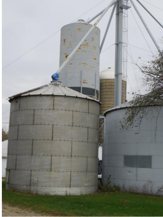
This photo reflects the bins and grain dryer located next to the home to the south.
