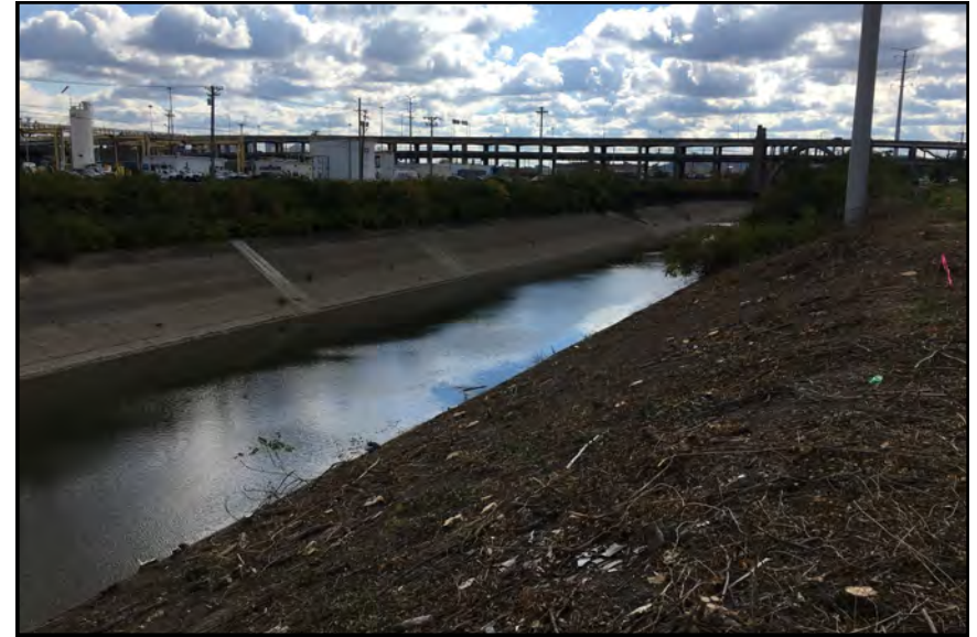
Photo 6. ROW Corridor, Mill Creek facing Southwest.
