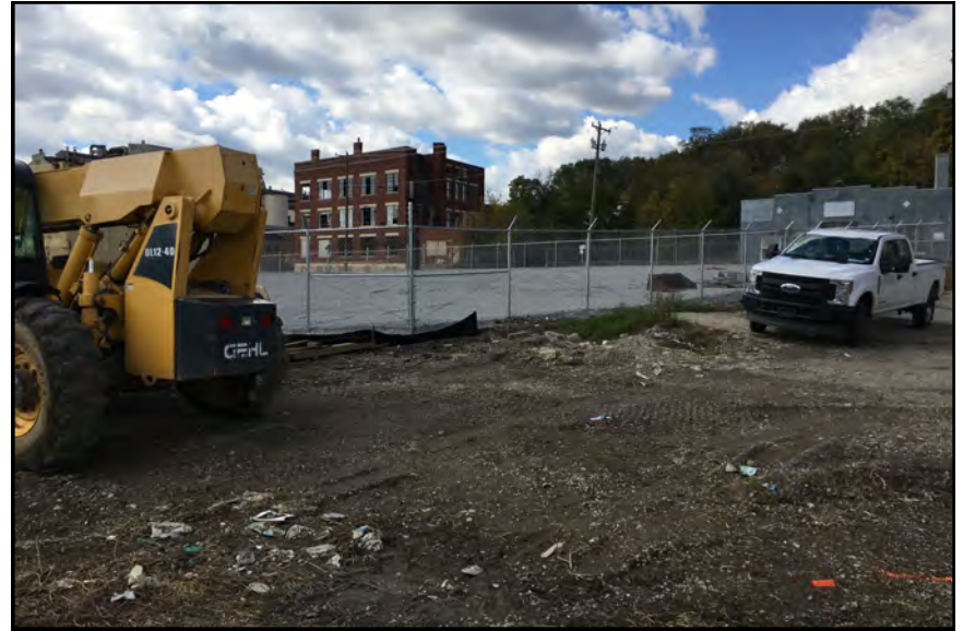
Photo 2. ROW Corridor, Near Pole HL19A, Duke Substation, facing Northwest.
