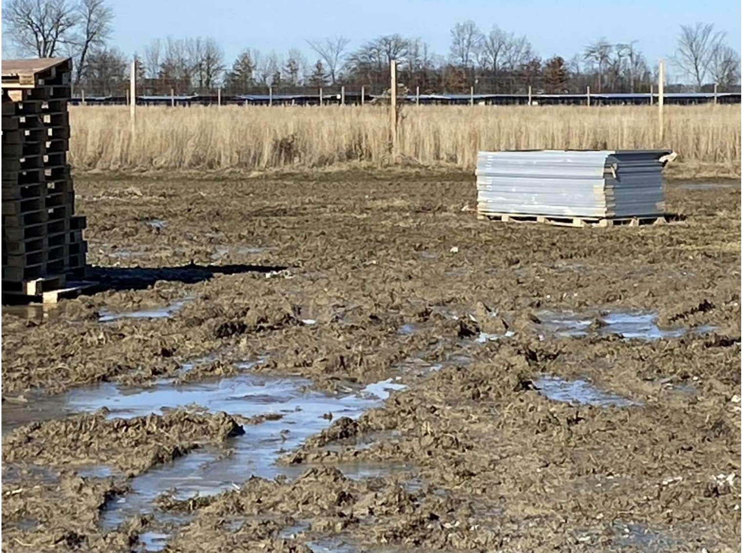
Photo 1: Example of material improperly stored in the middle of an un-stabilized area.
