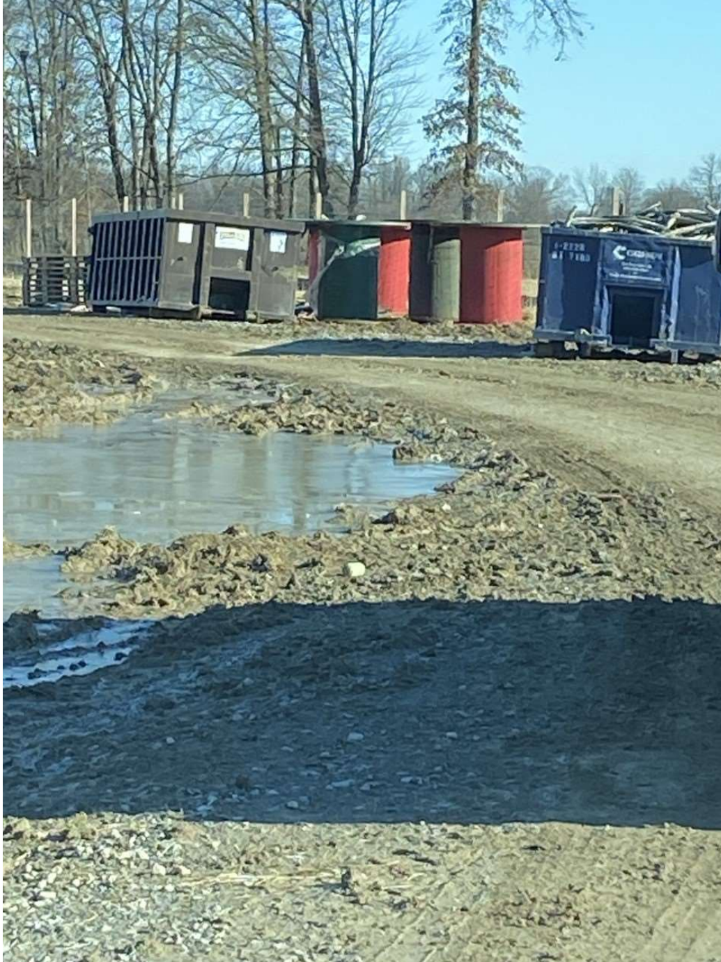
Photo3: Dumpsters and material stored on un-stabilized ground.
