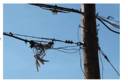
This photo from Emery Road, Warrensville Heights, OH, shows unsecured cable. The cable should be secured to the utility pole. The wind blows the unsecured service cable, damaging the copper inside the wire and causing service issues. In addition, this cable is within reach of passersby, causing a public safety hazard.
