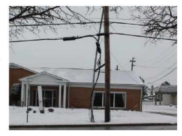
19. This photo from South Thomas. Road, Tallmadge Road, OH, shows a hanging pole, or a double-pole that has been cut before AT&T moved its facilities to the new pole. The old utility pole was cut with AT&T's terminal still attached to it. Left dangling, the old pole strains the cables and endangers the public. It is a service, worker, and public safety concern.
