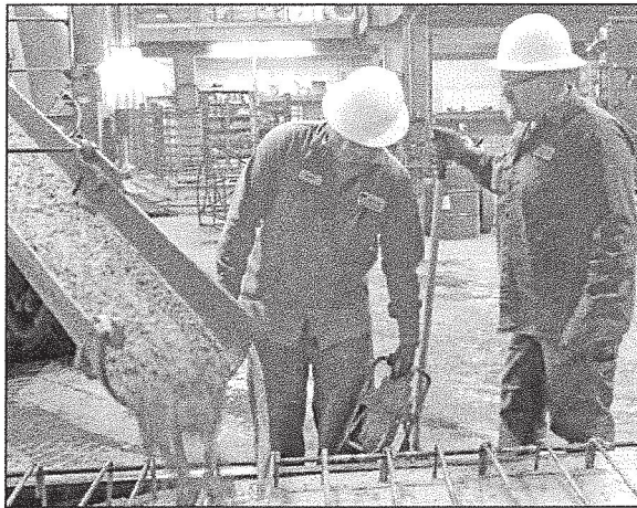
Bridge crew members with the Auglaize County Engineer spent time this week pouring concrete beams for bridge work in Wayne Township. The existing bridge is a concrete beam bridge on reinforced concrete abutments and has a span of 27 feet 10 inches with an overall beam length of 31 feet. Several beams on the bridge are due to be replaced. A total of nine beams were cast for the project.
