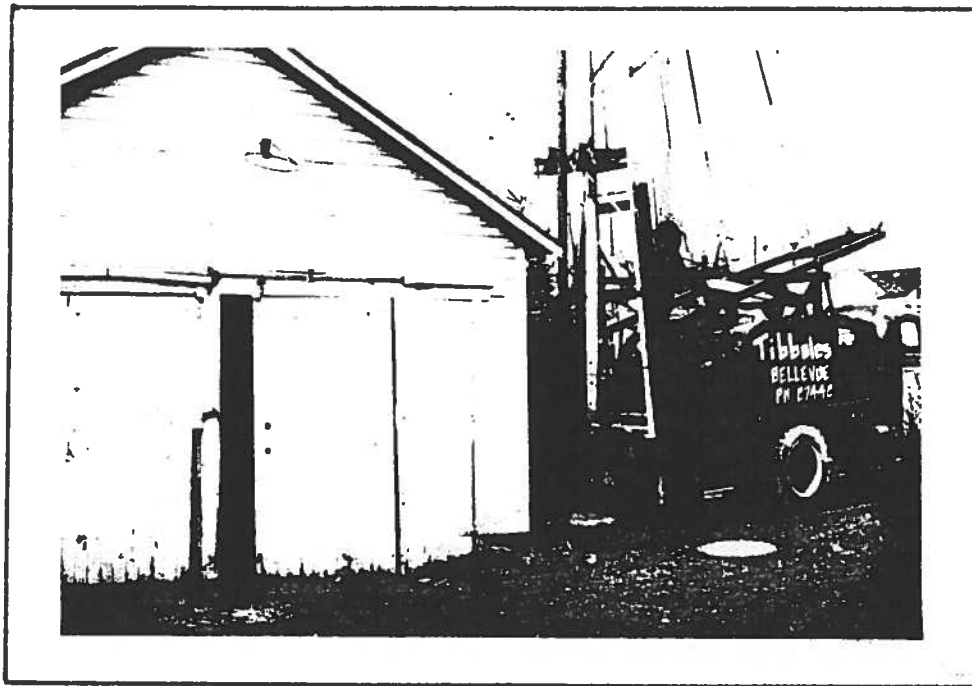
Household sewage has clogged this disposal well. Re-drilling will again permit free flow into the underlying limestone formations.
