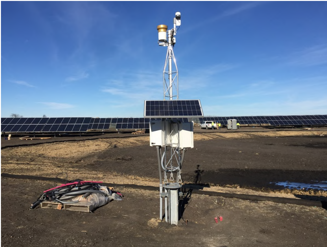
Inset 03-7. Representative Weather Station
