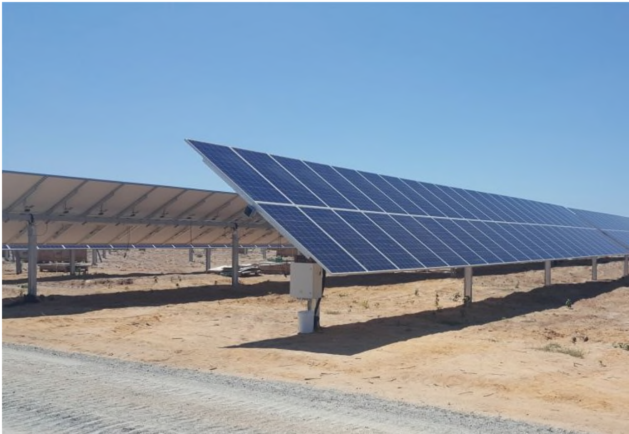
Inset 03-2. Representative Panel and Tracking Rack System
