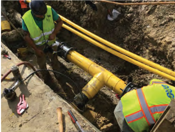
The tie-in on the north side of the circle.
