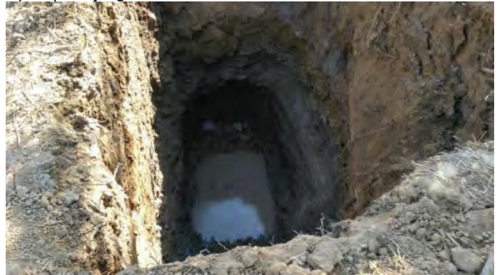
Open pit, trying to find bore head.
