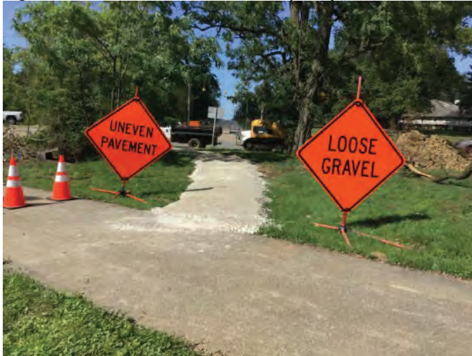
Signs erected at both ends of the temporary walk.
