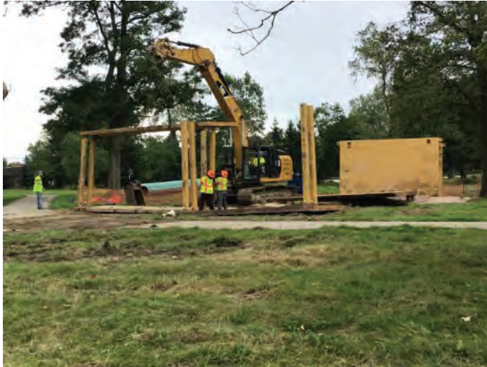
DRS putting together a trench box.
