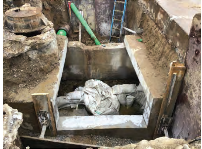
Culvert SAW CUT concrete
