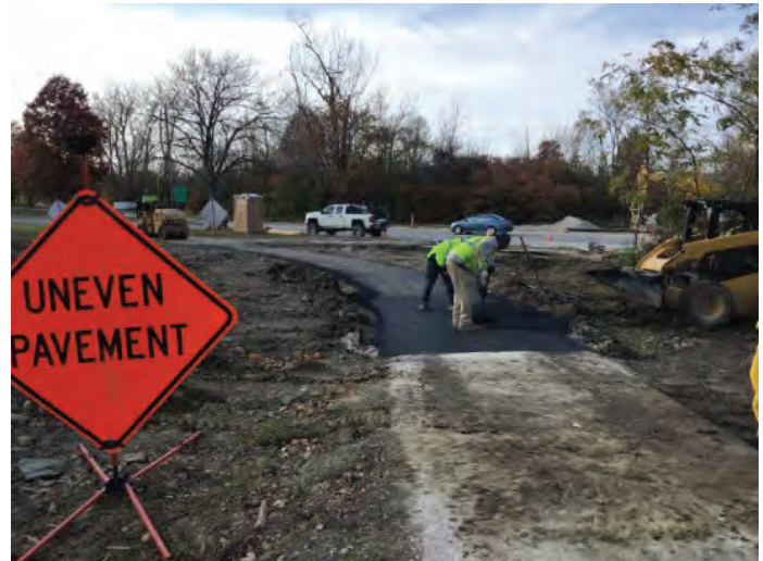
Sidewalk asphalt crew work inside the circle in front of Brainard Rd
