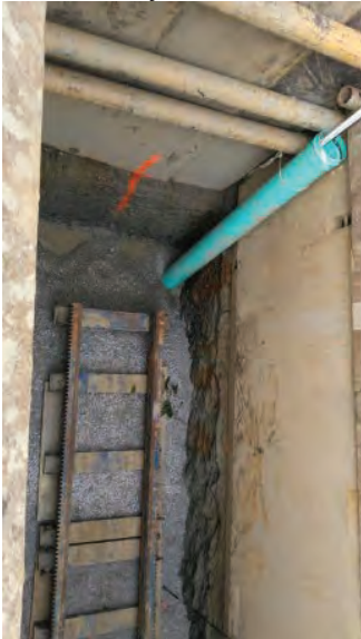
Tracks ready at bottom of bore pit.
