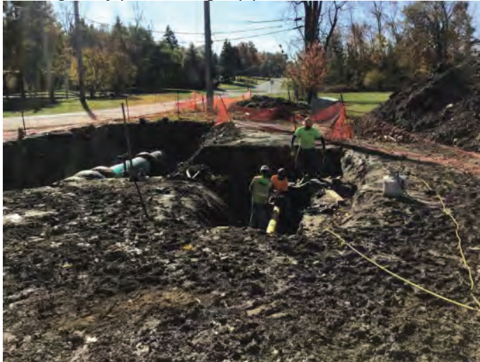
Working on by-pass main gas pipeline
