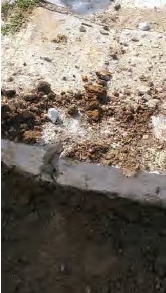
Sidewalk cut. Creaked Concrete apron.
