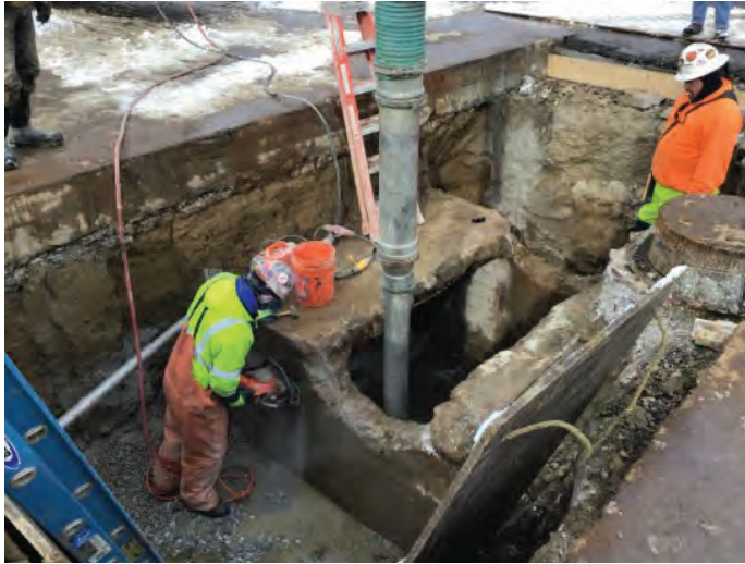
Saw cut concrete work
