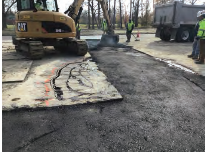
Work on the asphalt add second layer
