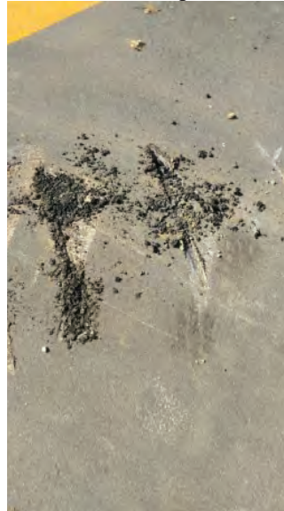
Some road damage from the excavator. Road was sweep
