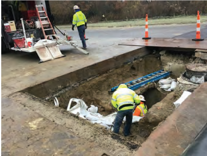
Work on saw cut concrete Culvert
