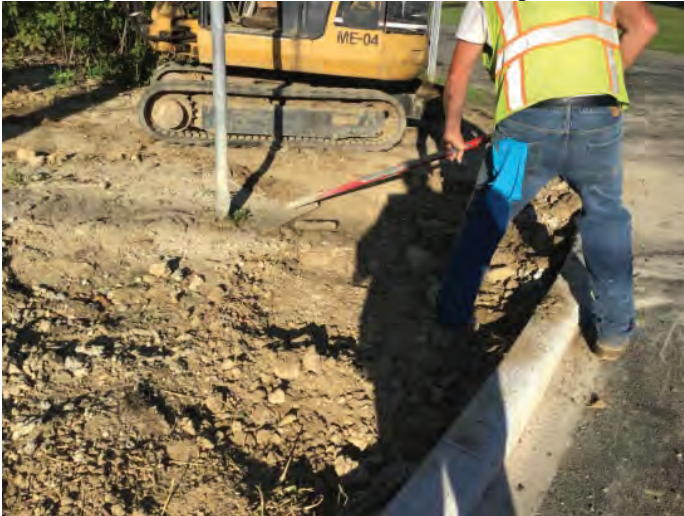
Backfilling behind the curb at Brainard and Belgrave.
