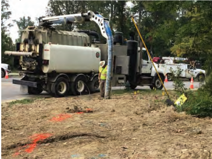
DRS pot holing to locate the water main.
