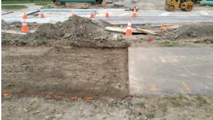
Bike path clear out ready for asphalt
