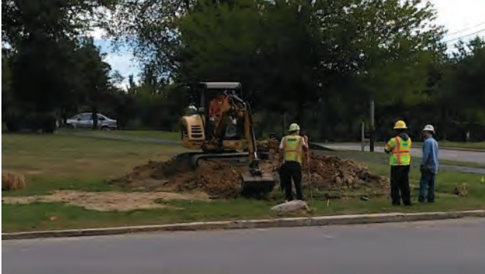
Backfilling on corner of Brainard and shaker
