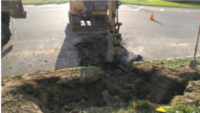
Pulling out road asphalt.
