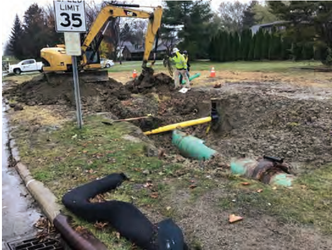
Excavated work on connection drain pipeline
