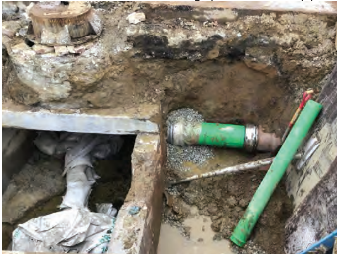
Culvert SAW CUT concrete & change part of the drain pipe
