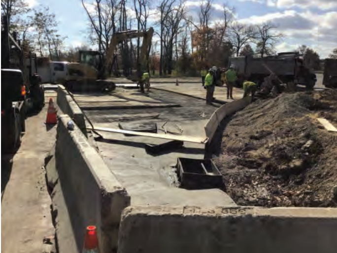
Work on the site new concrete curb and paving the road
