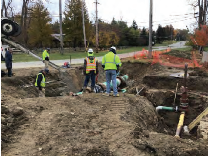
Delivered LSM200 to support main gas valve 4 yd
