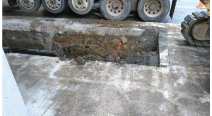
Cut concrete and enlarged pit under the bridge.
