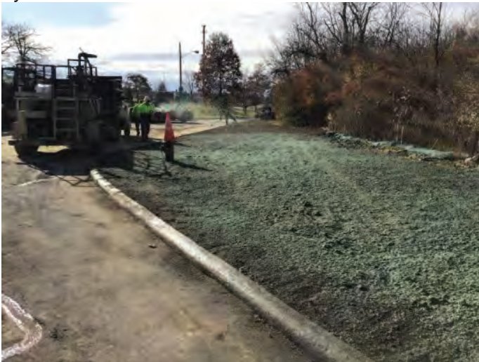
Hydro seeder and restoration work
