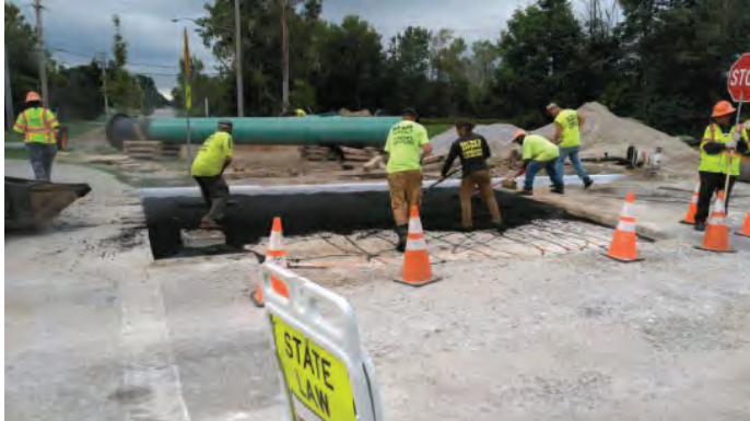
Laying asphalt First layer
