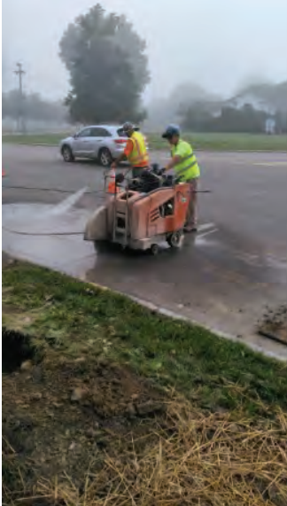
Cut crew cutting asphalt road.
