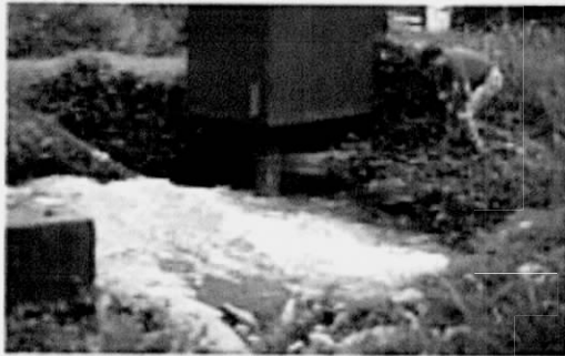
Fig. 36. (Below) This sinkhole has been modified to drain storm-water runoff. Two drainage wells have been drilled into the floor of the sinkhole. Rocks and hemispher- ical metal grates provide some filtration of sediments and organic debris.
