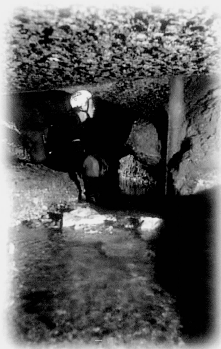
Fig. 50. Possible contaminants at higher elevations cannot directly reach the well because of the casing, but the well draws water from a cave stream that is exceptionally vulnerable to contamination.
