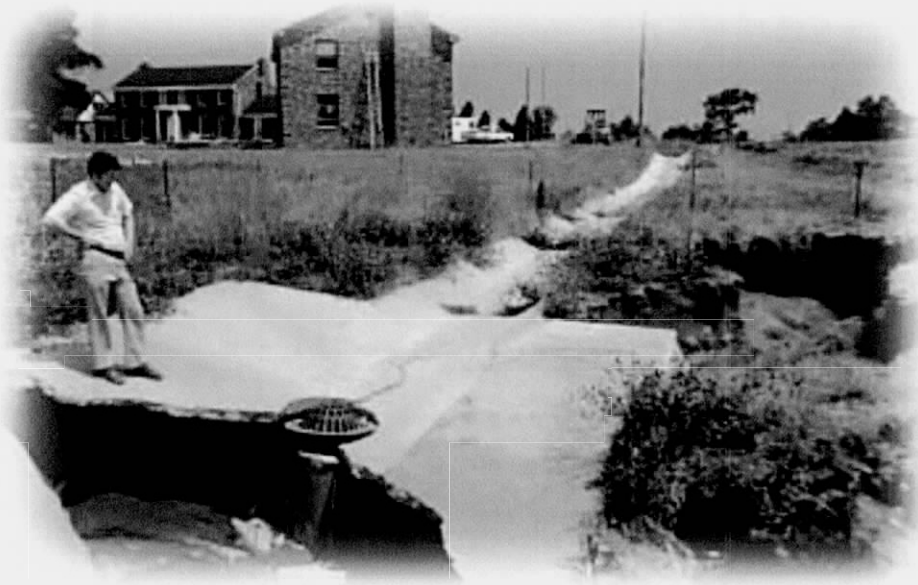
Fig. 30. Sinkhole collapse commonly results where the casings of drainage wells are not properly sealed to the bedrock.
