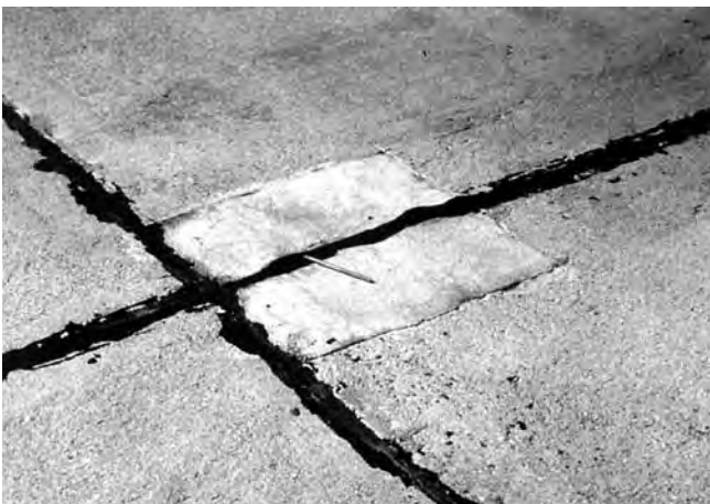
FIG. X2.28 Low-Severity Patching, Small
