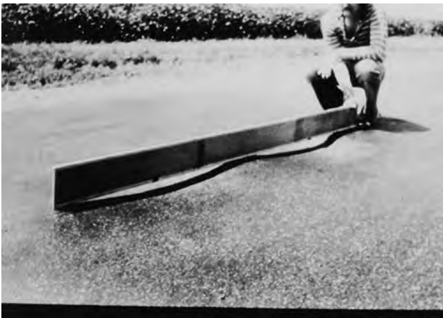
FIG. X1.15 High-Severity Corrugation
