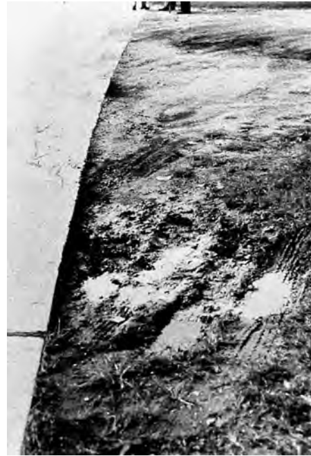
FIG. X2.20 Medium-Severity Lane/Shoulder Drop-Off
