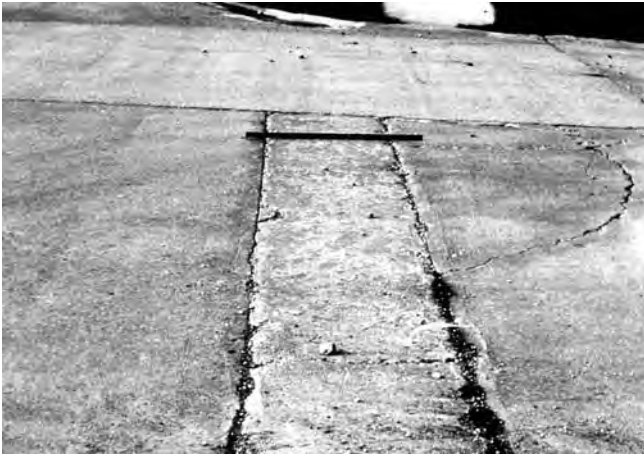
FIG. X2.26 Medium-Severity Patching, Large and Utility Cuts
