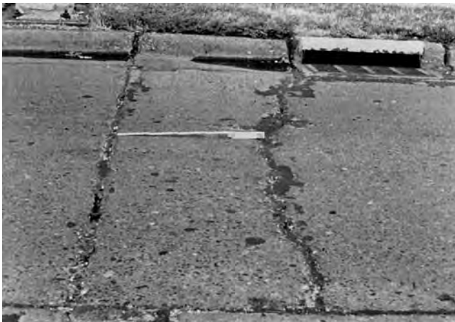
FIG. X2.35 Low-Severity Punchout
