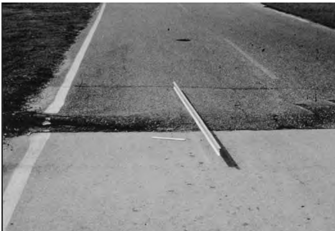
FIG. X1.46 High-Severity Shoving
