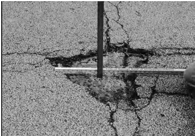
FIG. X1.36 Medium-Severity Pothole
