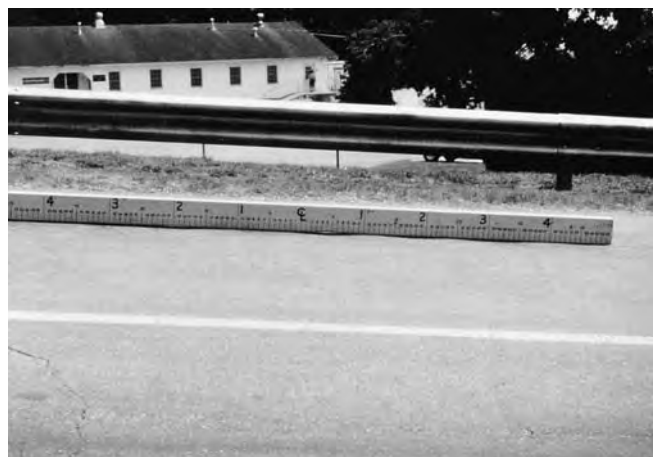
FIG. X1.13 Low-Severity Corrugation
