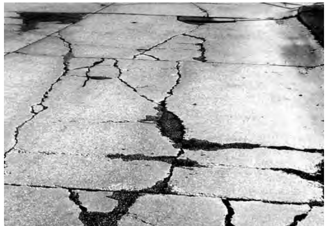
FIG. X2.9 High-Severity Divided Slab
