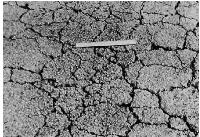
FIG. X1.3 High-Severity Alligator Cracking
