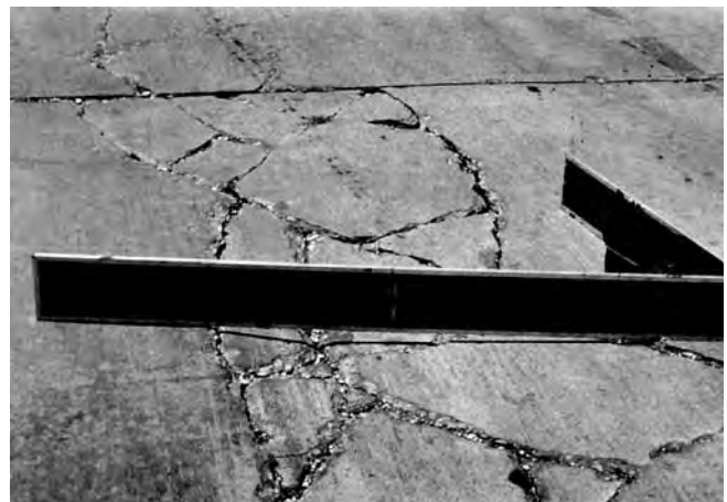
FIG. X2.37 High-Severity Punchout
