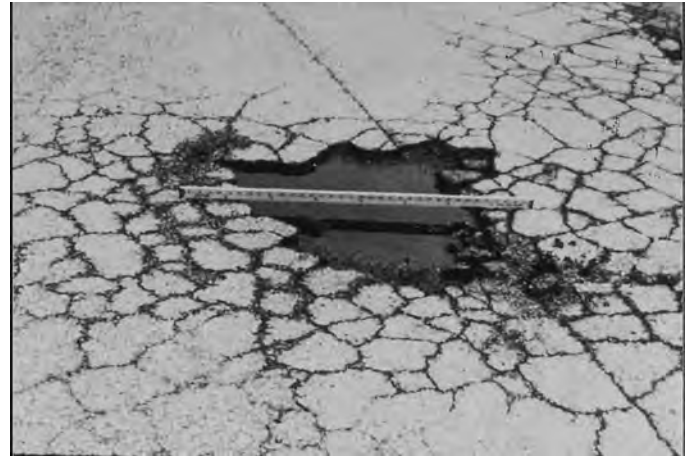
FIG. X1.37 High-Severity Pothole
