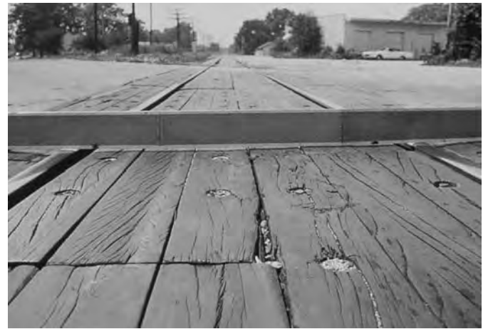
FIG. X1.38 Low-Severity Railroad Crossing
