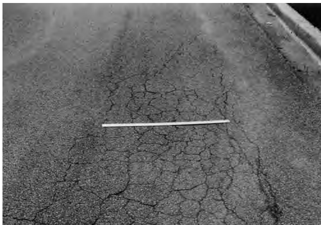
FIG. X1.2 Medium-Severity Alligator Cracking
