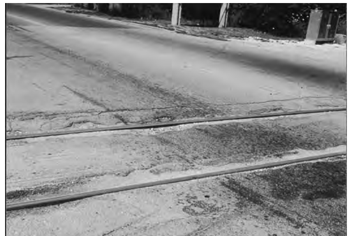
FIG. X1.39 Medium-Severity Railroad Crossing
