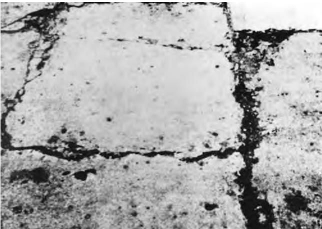
FIG. X2.27 High-Severity Patching, Large and Utility Cuts
