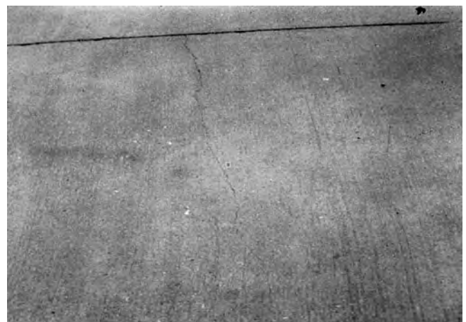
FIG. X2.44 Shrinkage Cracks
