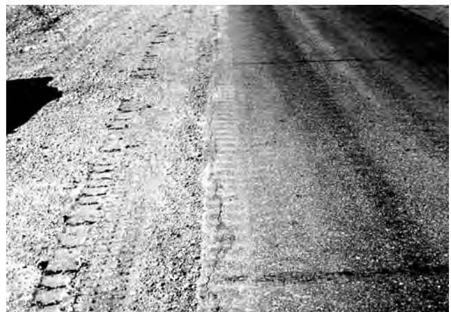
FIG. X1.22 Low-Severity Joint Reflection Cracking
