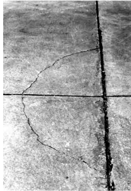
FIG. X2.4 Low-Severity Corner Break
