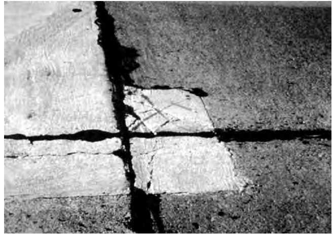
FIG. X2.29 Medium-Severity Patching, Small
