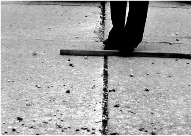
FIG. X2.13 Low-Severity Faulting
