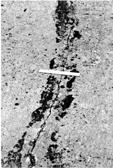
FIG. X2.22 Low-Severity Linear Cracking
