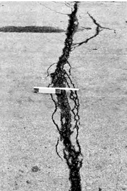
FIG. X1.24 High-Severity Joint Reflection Cracking
