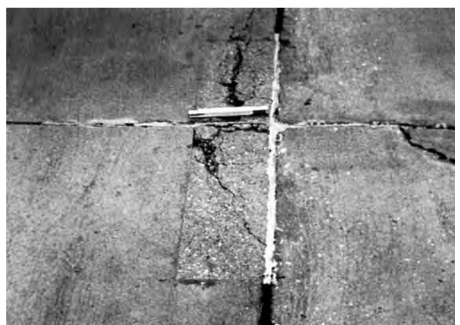
FIG. X2.30 High-Severity Patching, Small
