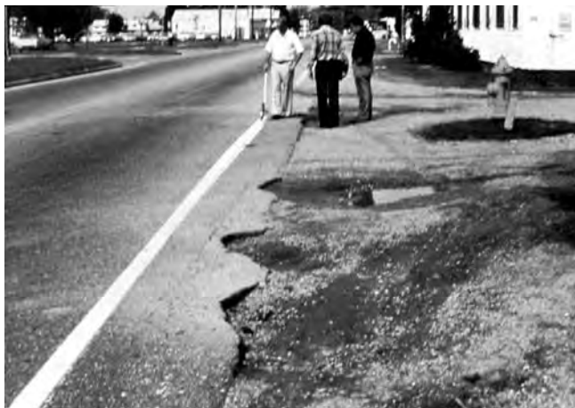
FIG. X1.21 High-Severity Edge Cracking
