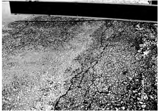
FIG. X1.12 High-Severity Bumps and Sags
