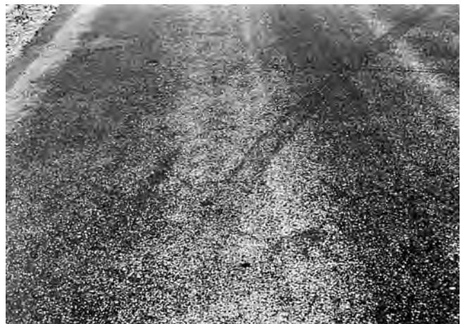
FIG. X1.4 Low-Severity Bleeding
