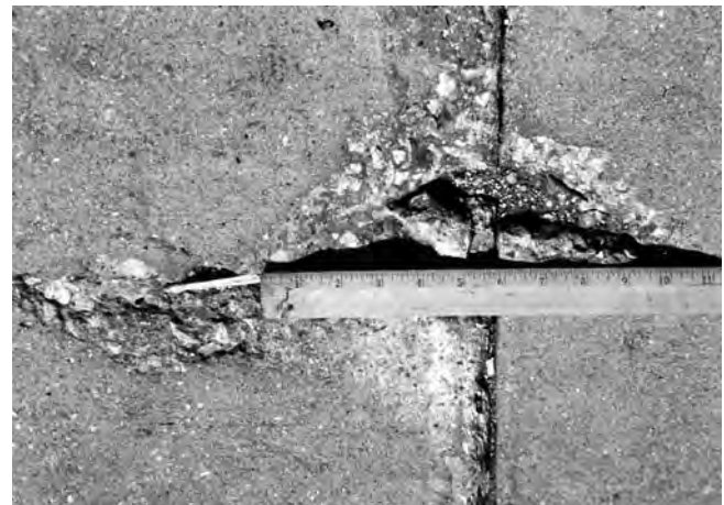
FIG. X2.46 Medium-Severity Spalling, Corner
