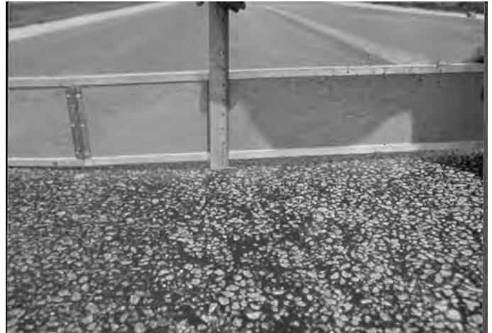
FIG. X1.42 Medium-Severity Rutting
