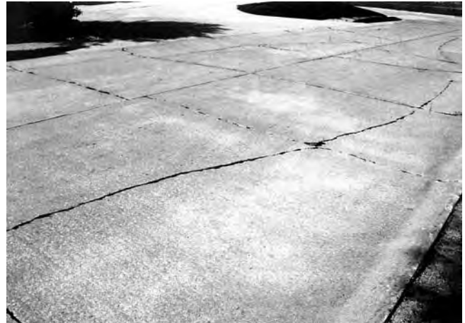
FIG. X2.7 Low-Severity Divided Slab
