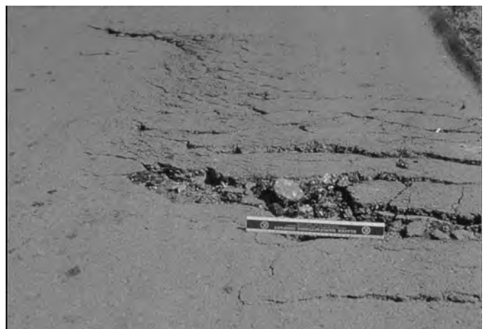
FIG. X1.49 High-Severity Slippage Cracking
