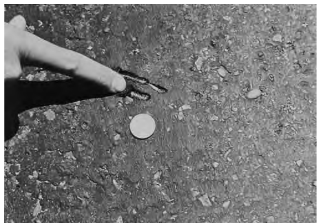
FIG. X1.5 Medium-Severity Bleeding
