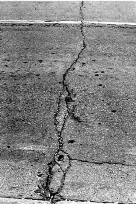
FIG. X1.23 Medium-Severity Joint Reflection Cracking
