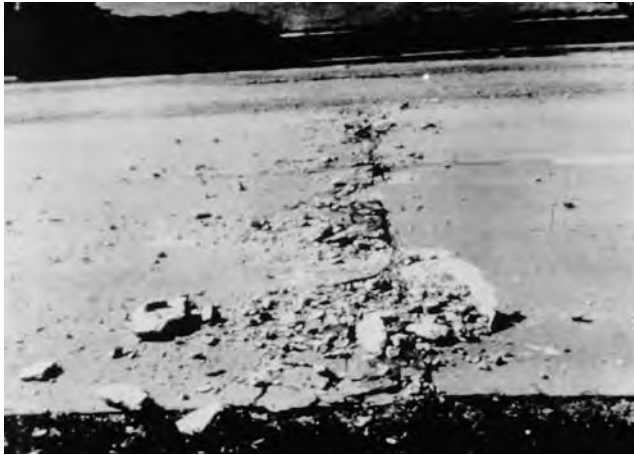
FIG. X2.2 Medium Severity Blowup/Buckling
