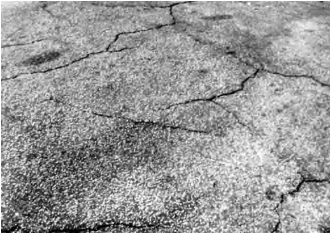
FIG. X1.9 High-Severity Block Cracking
