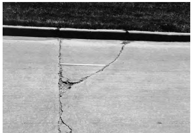
FIG. X2.5 Medium-Severity Corner Break
