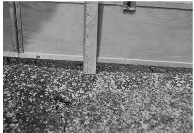
FIG. X1.43 High-Severity Rutting
