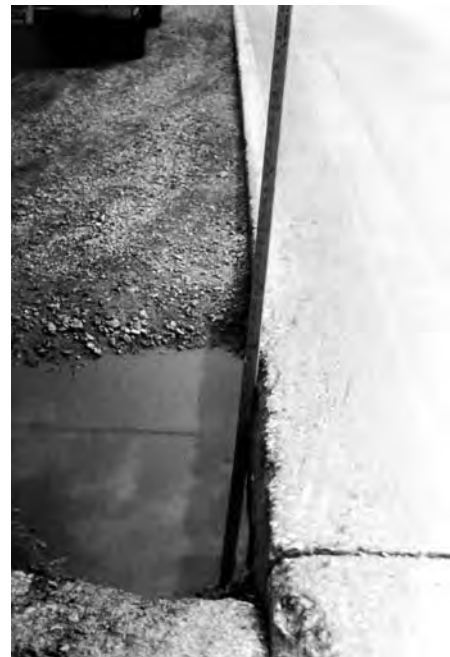
FIG. X2.21 High-Severity Lane/Shoulder Drop-Off
