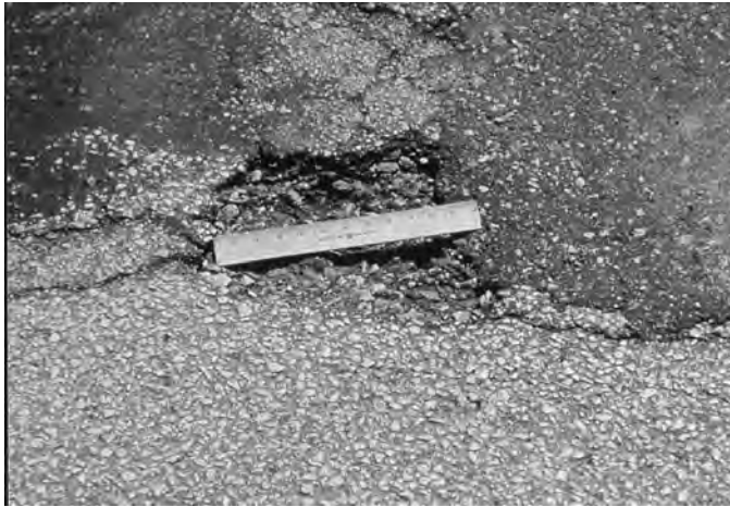
FIG. X1.35 Low-Severity Pothole
