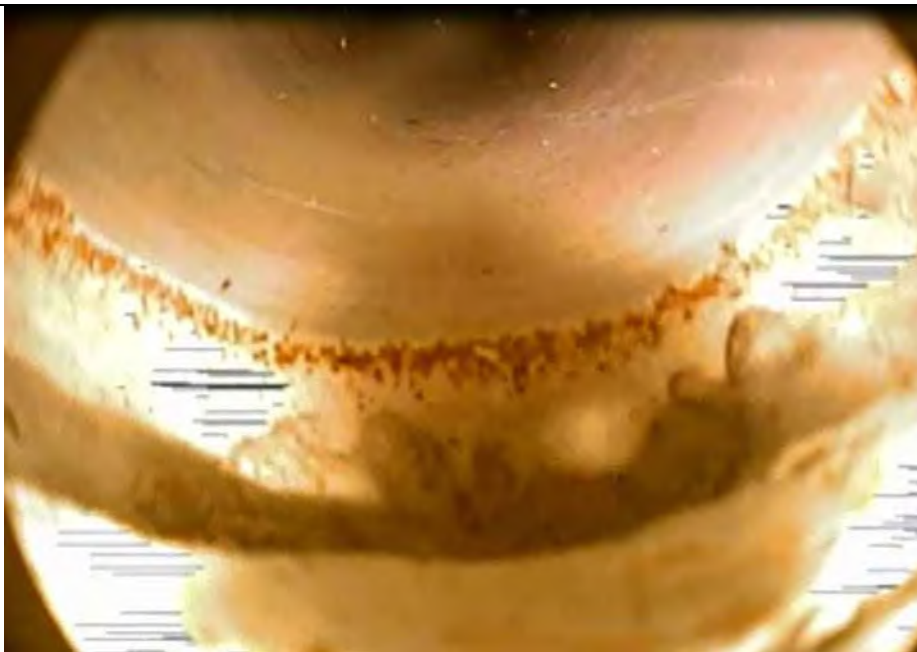
GEO-008, 6:28 33 ft, View of thin opening in sidewall, had back
