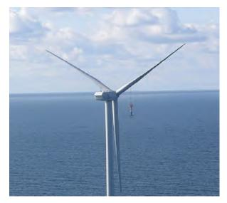
Fig. 15: Rotor in the "Y" position
