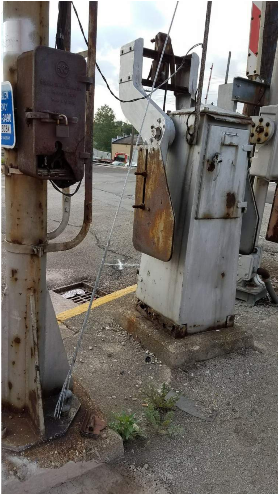
Broadway012 - Telecom Guy Wire Attached to Signal Foundation - NW QUAD looking East
