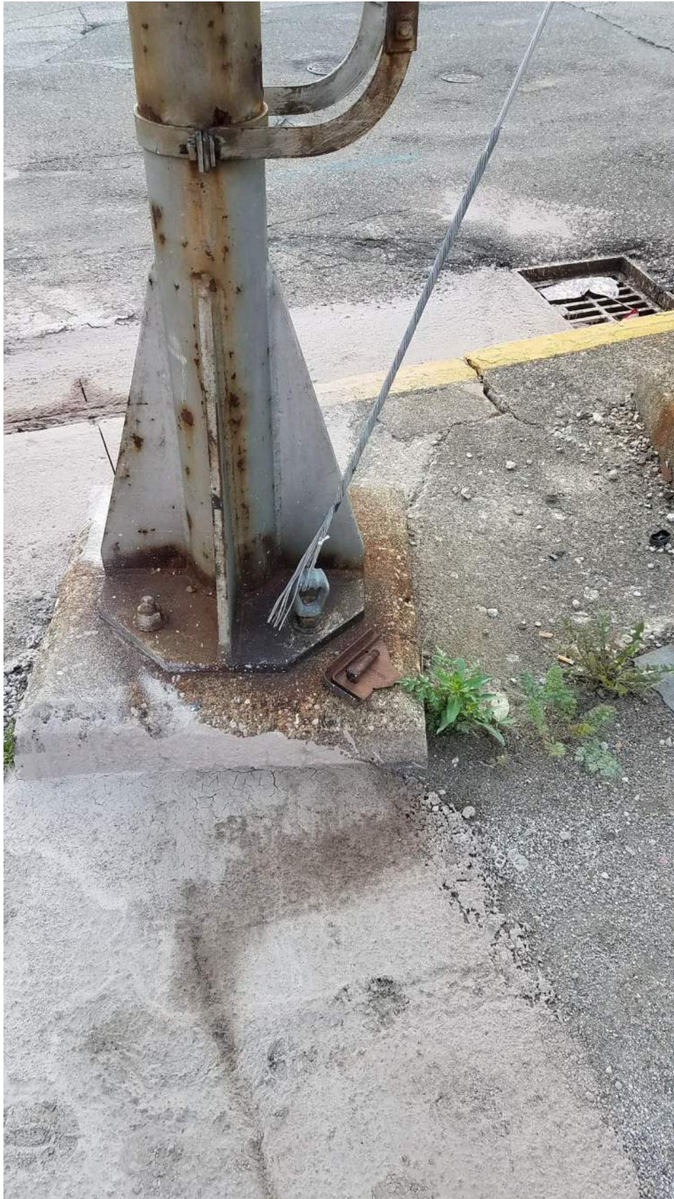
Broadway 011 - Telecom Guy Wire Attached to Signal Foundation - NW QUAD looking East
