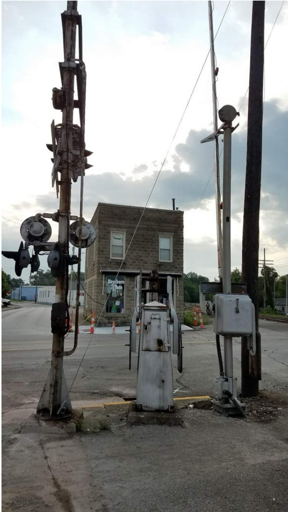
Broadway 010 - Existing Southbound Warning Devices, with Guy Wire Shown - NW QUAD looking East
