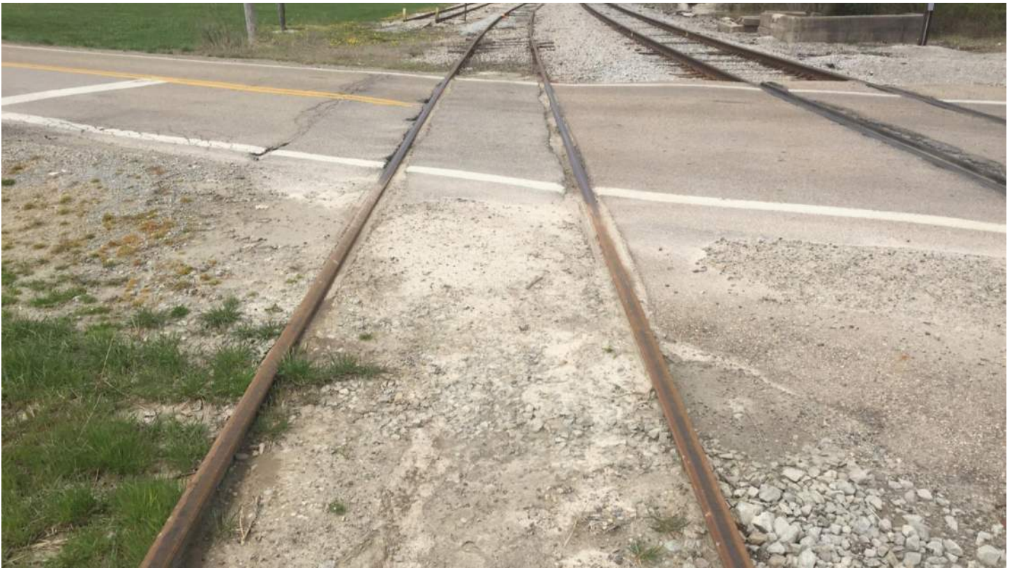
SR-55 002 – SR55 Crossing Surface and Fouled Siding Ballast – SE QUAD looking West
