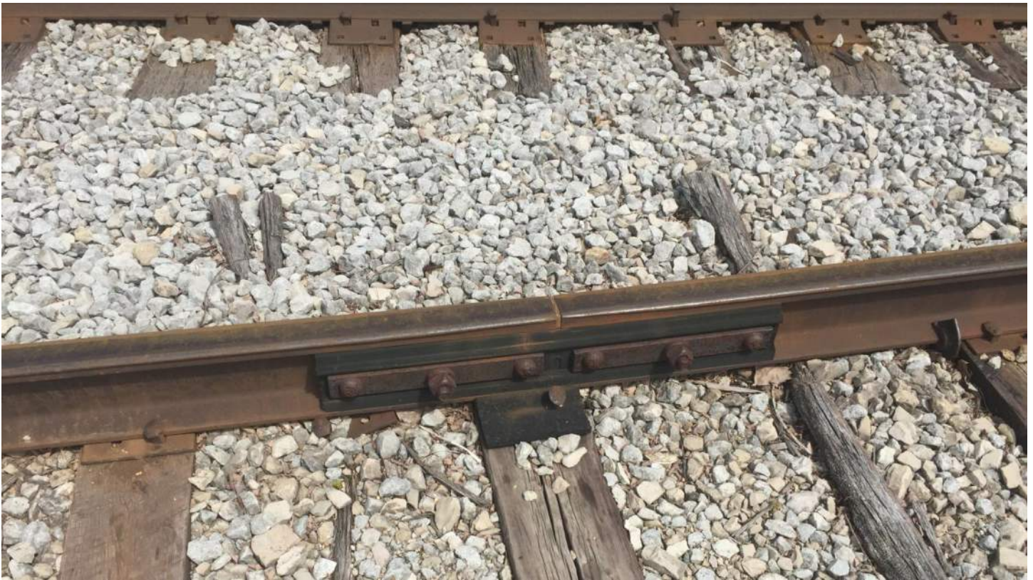
Hampton-Donnelsville 025 – Insulated Joint in Siding – SE QUAD looking North
