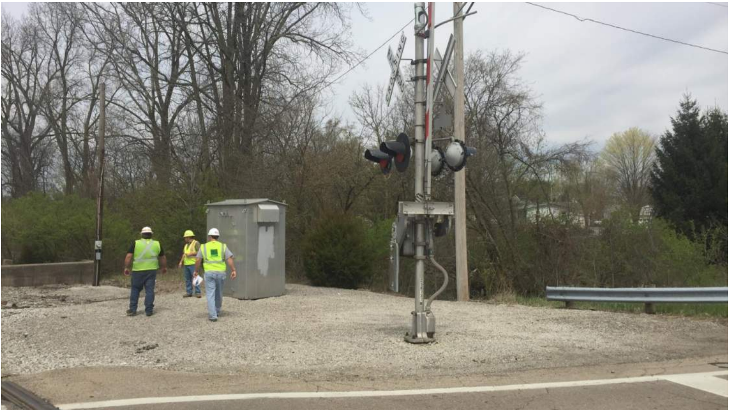
SR-55 004 – SR55 Signal Enclosure and Flashing Lights – NE QUAD looking West
