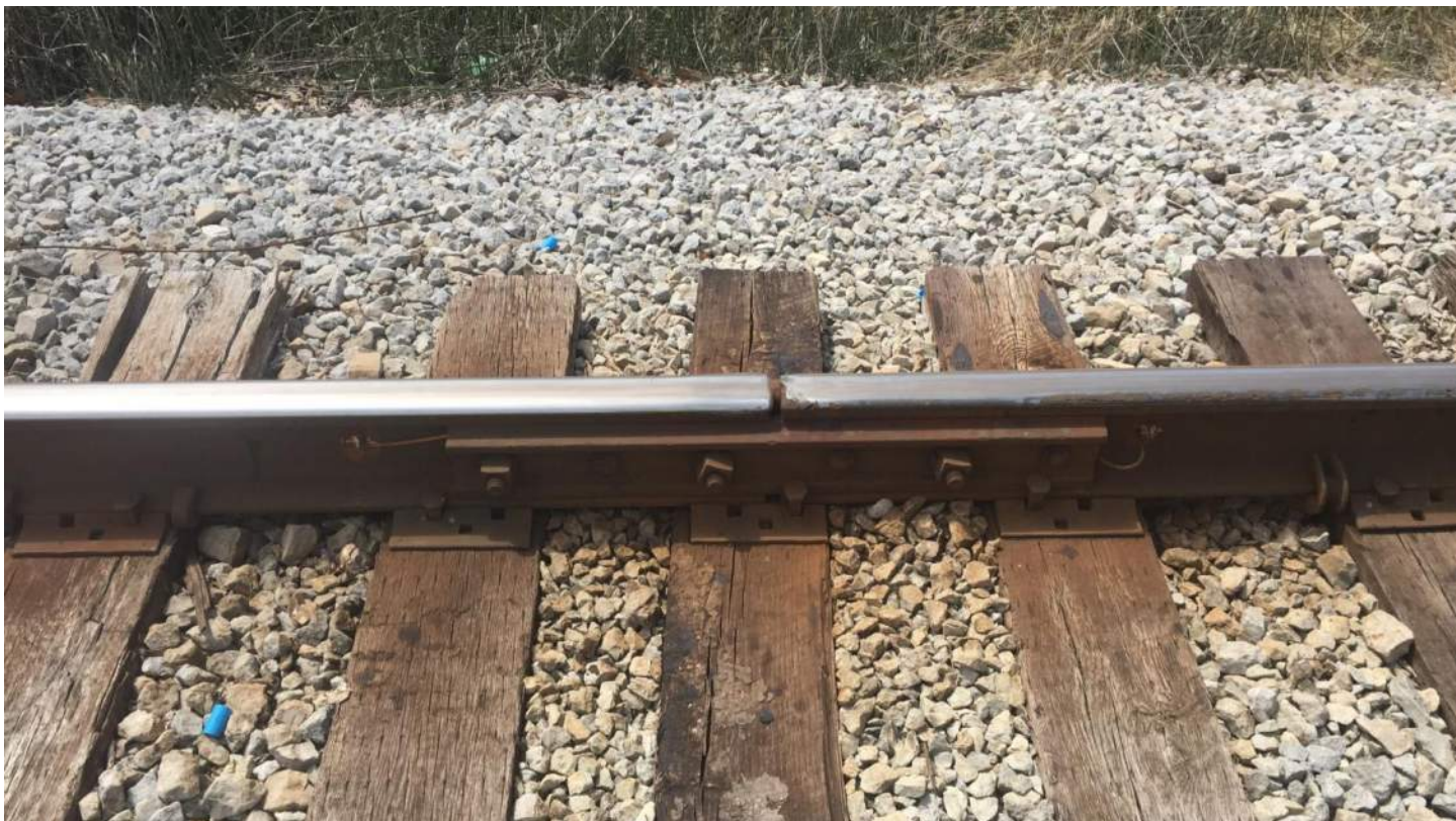
Hampton-Donnelsville 017 – Siding Joints – NE QUAD looking South
