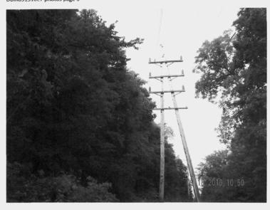
This photo was taken in the area of the Maple that grew into the line causing the damage. Note how close the trees are on the uphill or left side of the lines. Camera pointed west.
