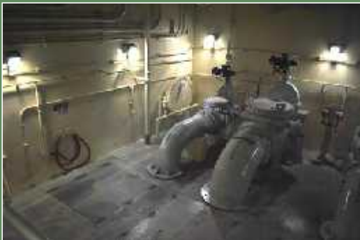
25-watt LEDtronics WWL12-8X2W-XPW-001 wall-paks replaced 250-watt HPS at Union Sanitation District's wastewater treatment plant in Union City, California
