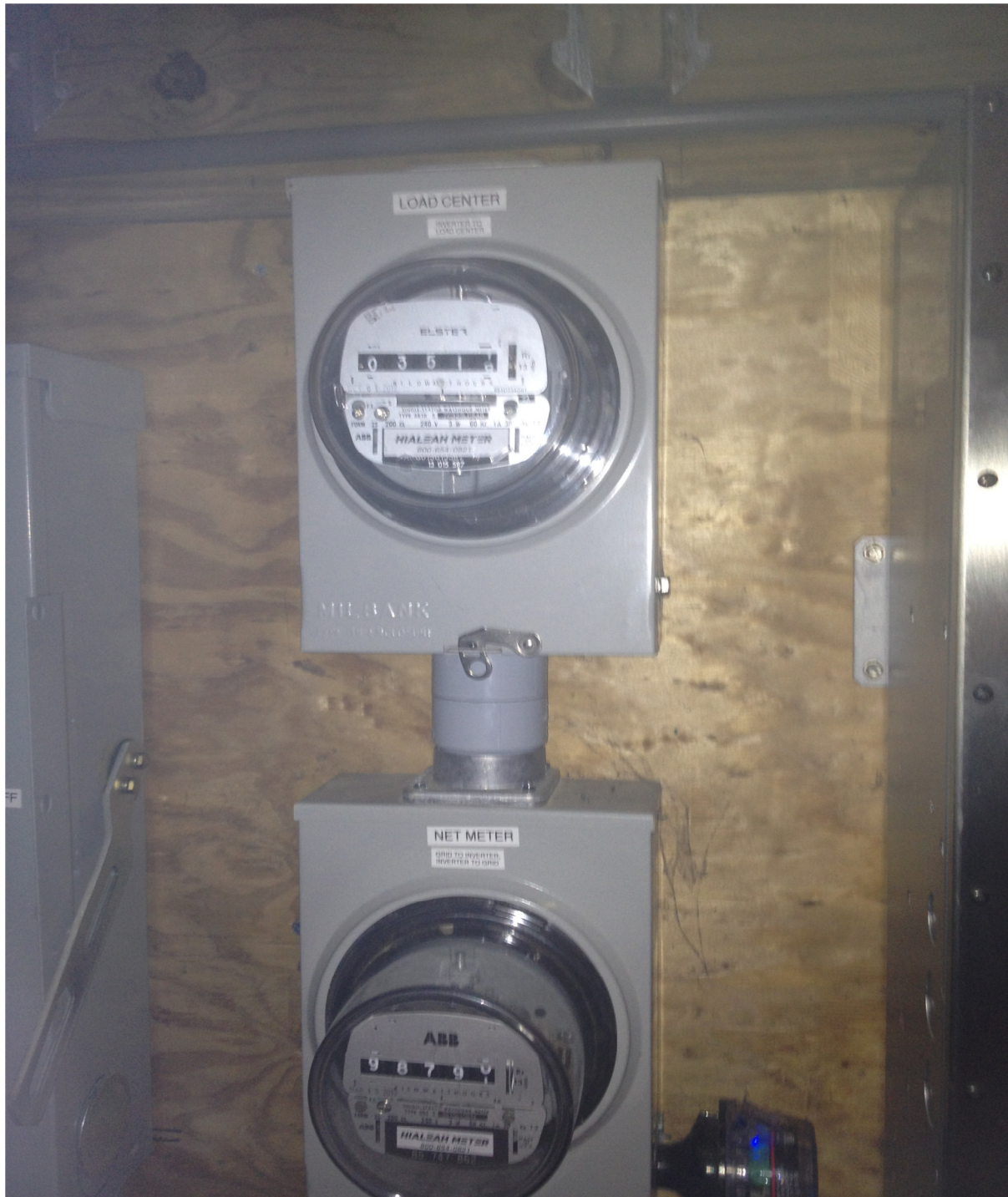
Photographs of Meters together Upper Meter is Loadcenter Meter, Lower is Net Meter
