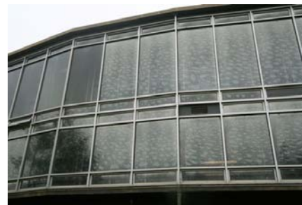
Failed window film treatment.
