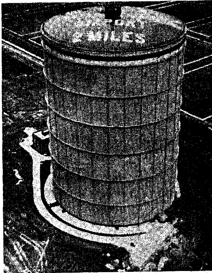
FIG. 16. Twenty Million Cubic Foot M. A. N. Waterless Holder of The Peoples Gas Light & Coke Company, Chicago, Ill. 283 ft. Diameter by 408 ft. High. (Courtesy of The Bartlett Hayward Company, Baltimore, Md.)
