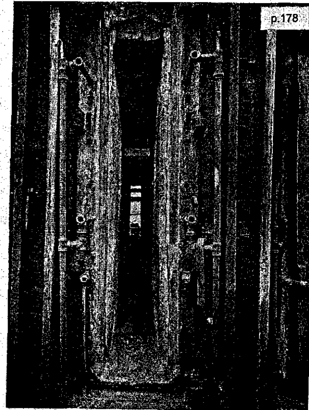
FIG. 58.—View Through Semet-Solvay By-Product Coke Oven, End to End, after 16 Years' Service.
