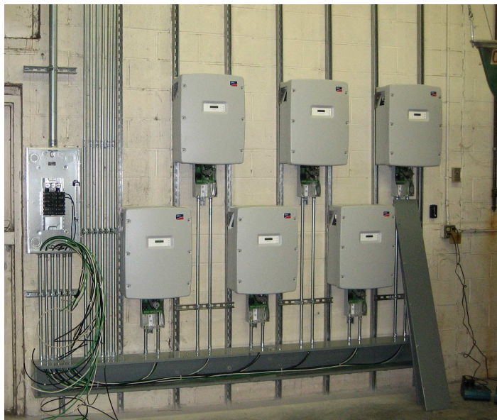
Inverters and breaker box (final wiring is now complete)
