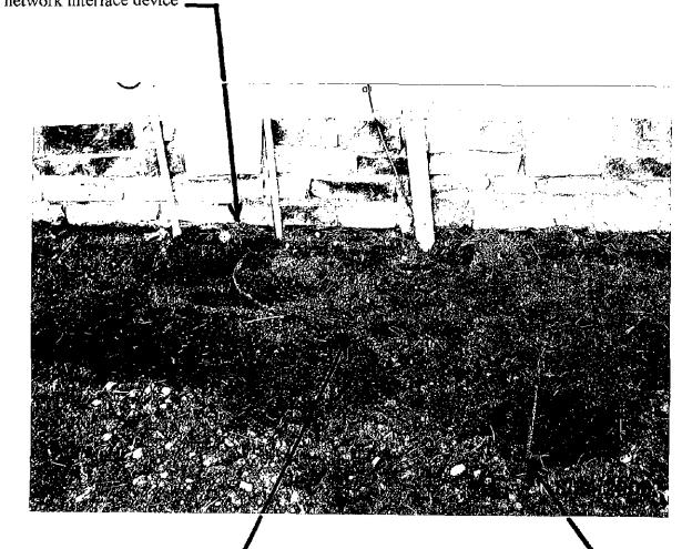
Cable travels just under the surface to the conduit Cable comes up out of the trench About 3 feet from the foundation.
