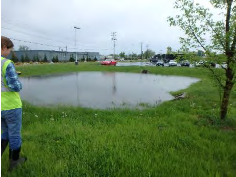
Photograph 17: Representative view of a detention pond within an industrial park.
